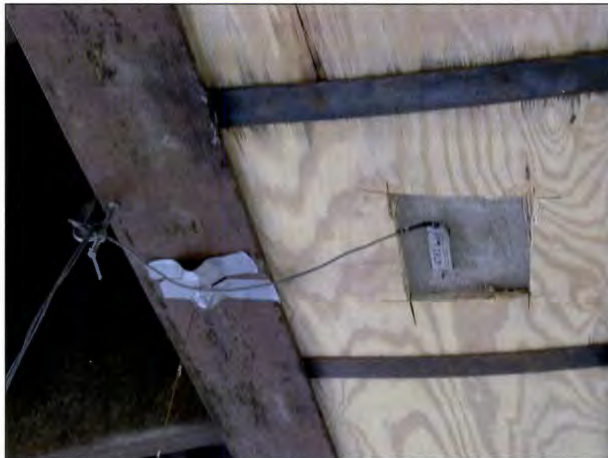
b. Strain transducer on the concrete LFC
