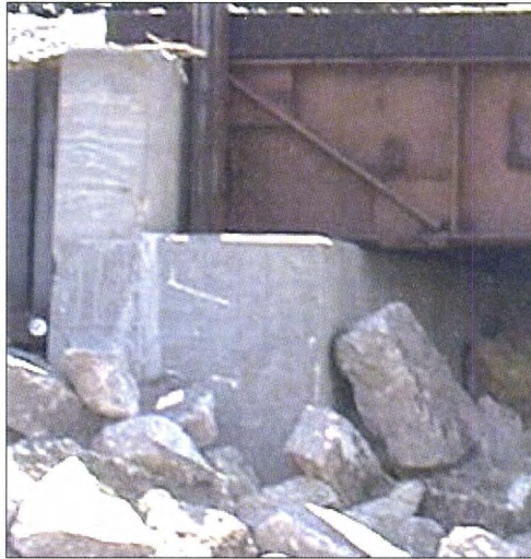
c. Side view of concrete abutment
