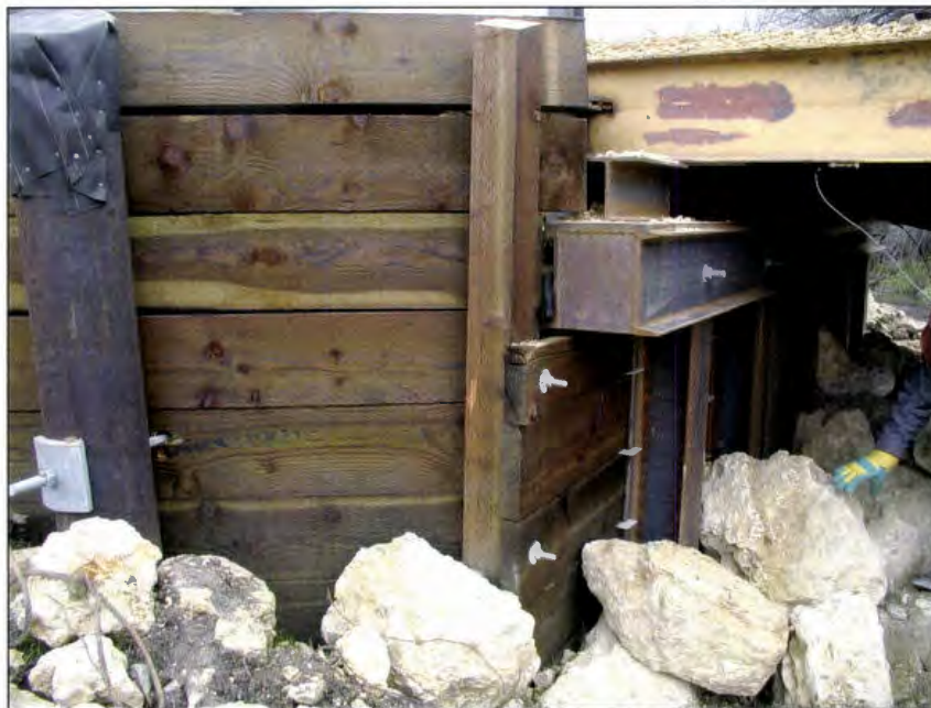
b. Photograph of wing wall and side view of cap beam
