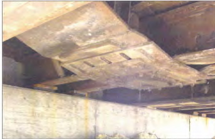
b. View of interior girder resting on abutment cap beam
