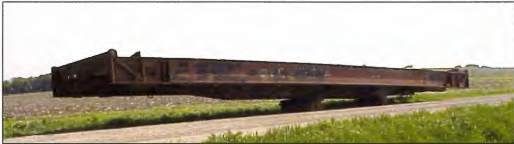
b. The 56-ft V-deck RRFC after trimming
