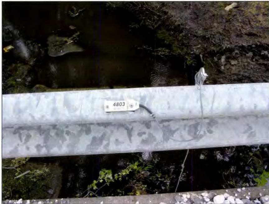
a. Strain transducer at midspan on the south guardrail
