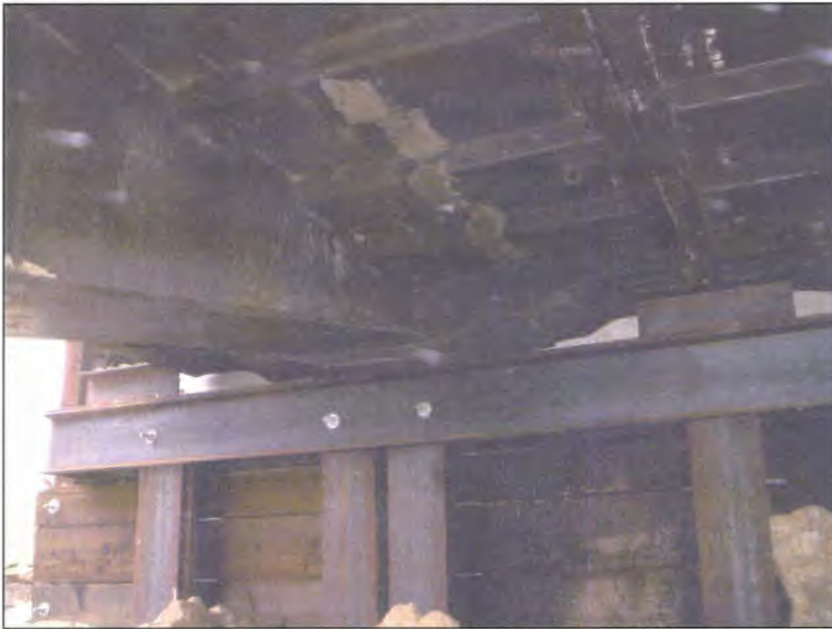
b. Photograph of abutment and backwall
